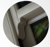
Run-through Sash Horns
