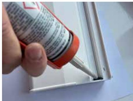
Then attach the sill end caps and add a layer of silicone in the channel to stop any drainage water from escaping down the side of the sill.
