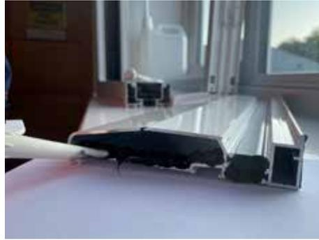
Before fixing the sill to the bottom of the aperture, fill the two outwards facing chambers (as illustrated) with a thick line of silicone along the edge. This is to stop any drainage water from escaping the drainage channels. Use an appropriate colour that matches the frame finish.
