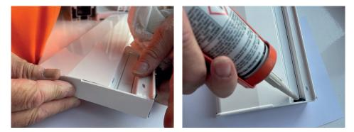
Then attach the sill end caps and add a layer of silicone in the channel to stop any drainage water form escaping down the side of the sill.
