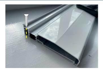
Fix the sill to the bottom of the aperture through the first inwards facing chamber as illustrated. No drainage will go through this chamber so you can go all the way through.
