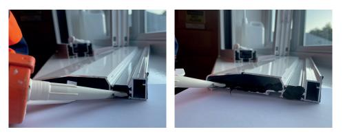
Before fixing the sill to the bottom of the aperture, fill the two outwards facing chambers (as illustrated) with a thick line of silicone along the edge. This is to stop any drainage water from escaping the drainge channels. Use an appropriate colour that matches the frame finish.
