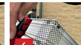
It is important that after the joint has been made to smother the outer corner where the cleat blocks fit to ensure no water ingress at the side and bottom.
